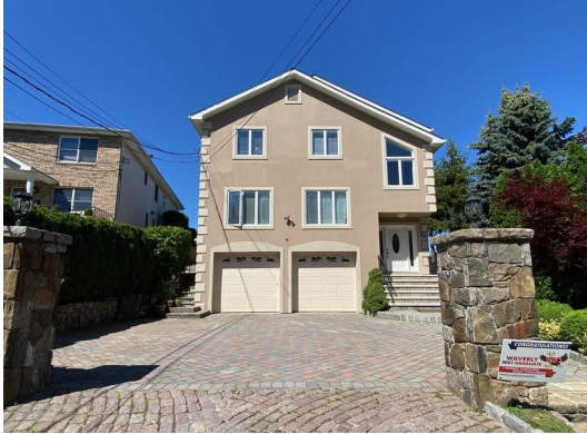
Exterior – 46 Glen Road
